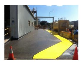
This large project included surface preparation of some 6,500sqm of concrete including expansion joints and construction joints followed by the application of a 3mm coating of Rhino PP1195 Pure Polyurea.
